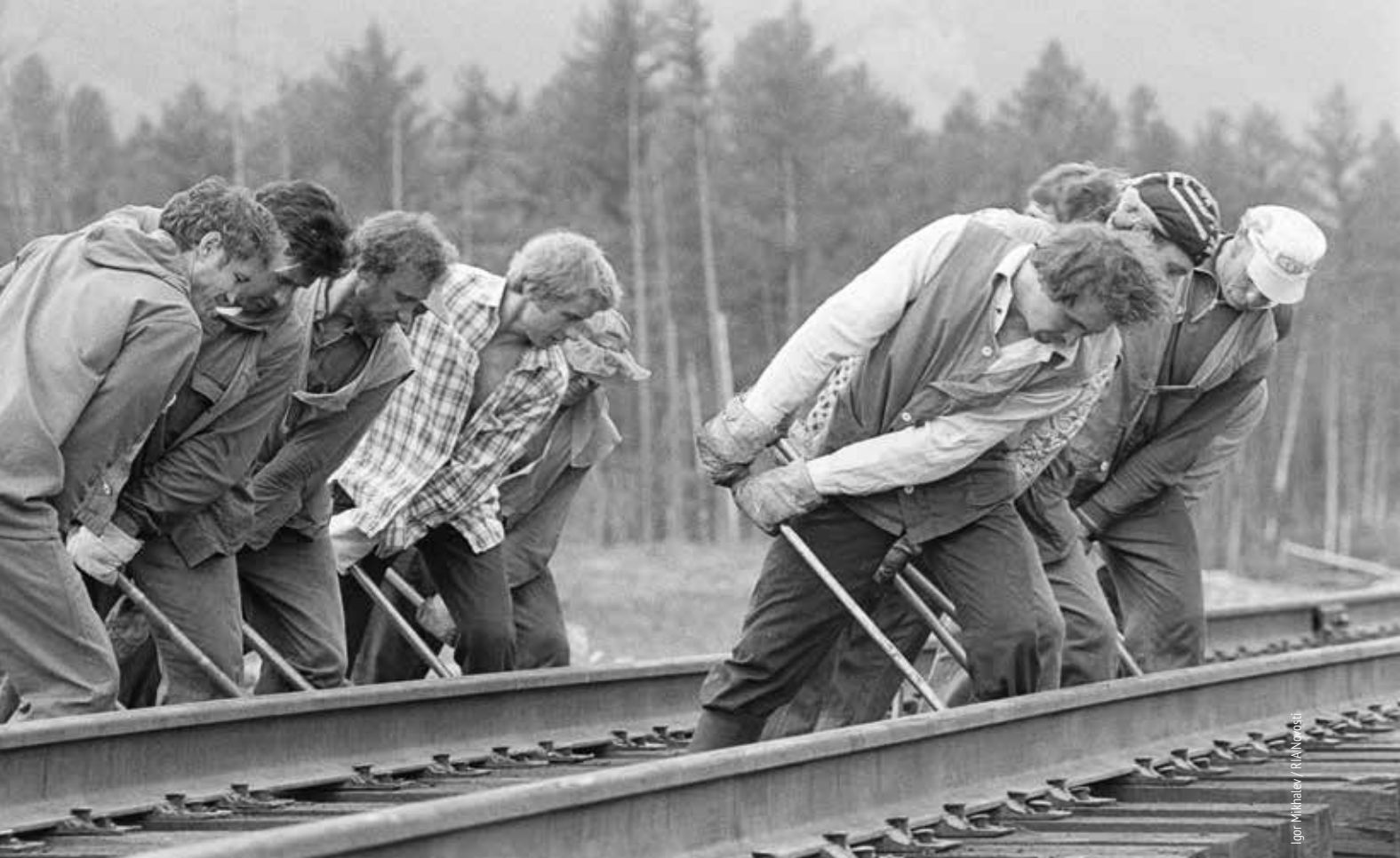
The photo depicts the laying of rails during construction of the Baikal-Amur railway
